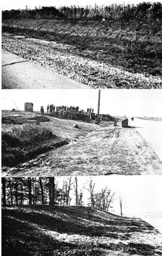
FIG. 18. Showing artificial changes in road margins. Top, example of original roadside condition; middle, showing the C.C.C. crew sloping the bank preparatory to planting; lower, a finished piece of roadside, after it has been graded and planted.
