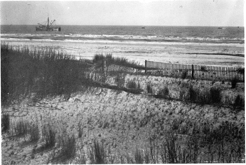
Fig. 2. Sand dune stabilization project at Sea Rim State Park, Jefferson County. Mechanical barriers promote capture of sand and provide favorable microhabitat for seedlings.
