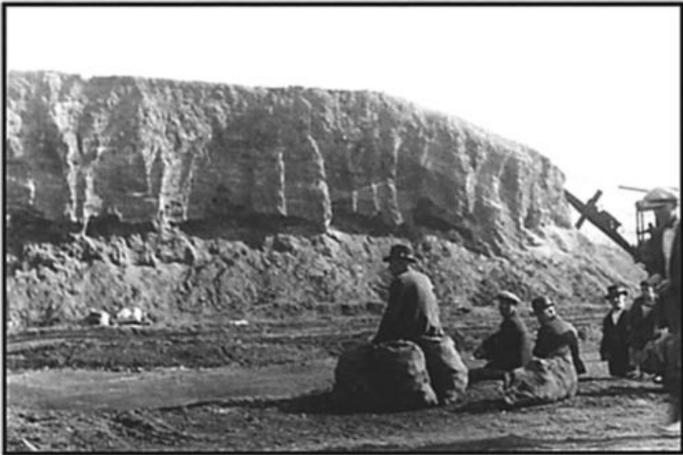
FIG. 2. Demolition of the Emeryville Shellmound by steam shovel, 1924. (Photo courtesy of the Phoebe A. Hearst Museum of Anthropology.)
