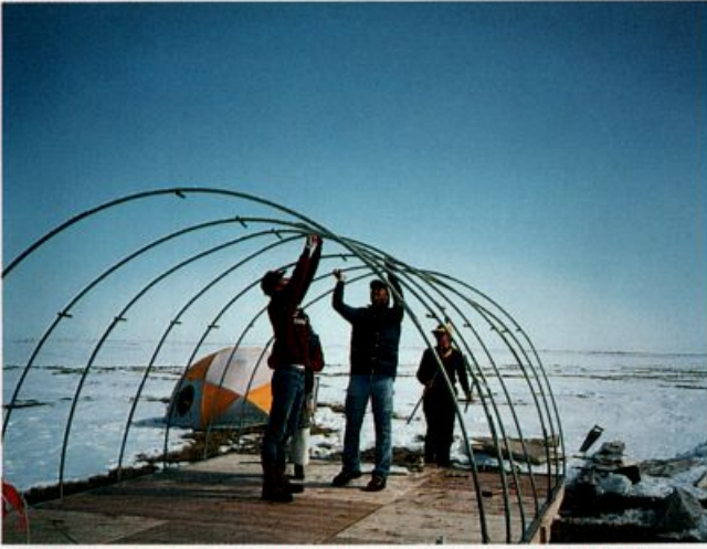
Building a weatherport in Alaska. Photograph/Pam Miller.
