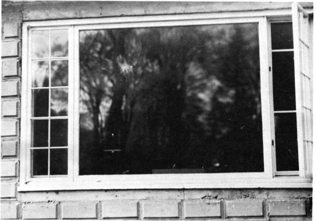
Window from outside
