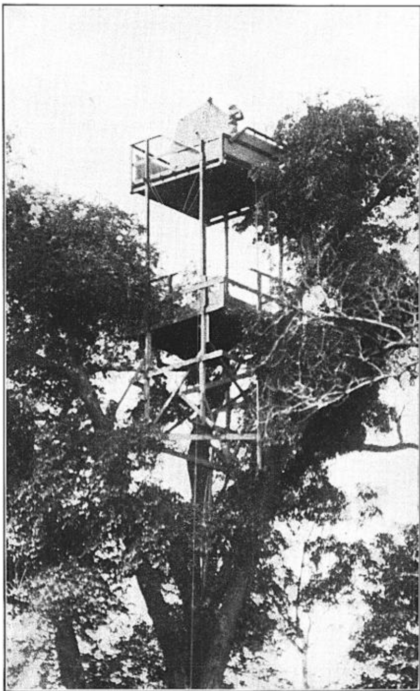
OBSERVATORY WITH SECOND PLATFORM ADDED IN 1923, 95 FT. FROM GROUND. STEEL LADDER PASSES FROM MAIN TRUNK THROUGH EACH PLATFORM.
