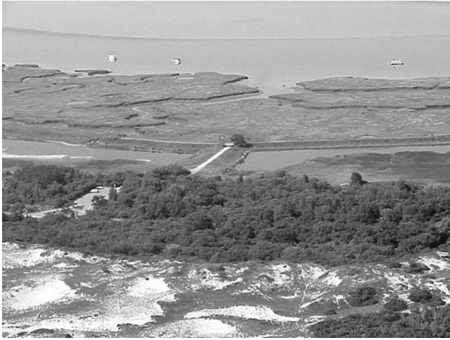
HELLCAT NATURE AREA SHOWING BILL FORWARD POOL (LEFT), NORTH POOL (RIGHT), DIKES, OBSERVATION PLATFORM (CENTER), AND PARKING LOT (LEFT) — AERIAL PHOTOGRAPH BY DAVID LARSON.
