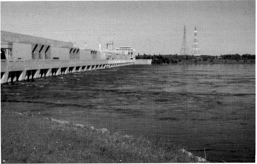
Figure 1: Moses/Saunders Power Dam. Photo by B.M. Di Labio.
