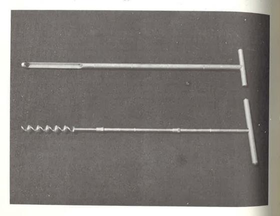
Soil sampling tube (above) and auger (below) used in setting net poles.
