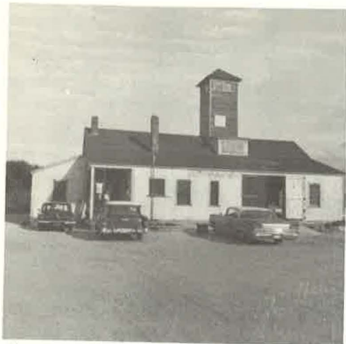
Left -- Headquarters at Island Beach Operation Recovery is an old Coast Guard Station
