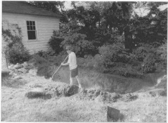
Figure 1. Excavation of the pond in progress, showing the basin and the shelf around the edge (photographs by the author)
