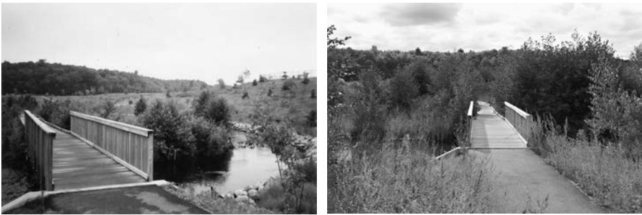
Figure 3: Boardwalk entrance to the project site. Left: 2004, Clark Ewer photograph; Right: September, 2005, John Marsh photograph.
