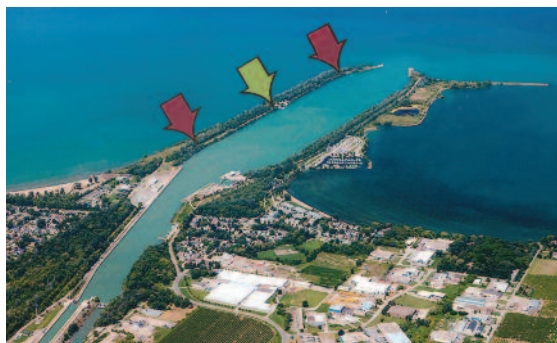
Figure 5. East and west piers of the Welland Canal exiting into Lake Ontario at Port Weller, St. Catharines. The red arrows pinpoint the areas on the west pier where cormorants are nesting, or attempted to nest. The green arrow identifies the location of the Canadian Coast Guard Station.
