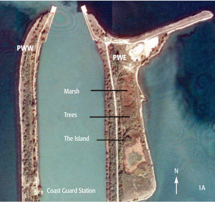
Figure 1A. The Piers, September 1995.
